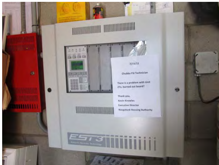
Fully addressable fire alarm control panel monitors and supervises hardwired end devices throughout the development
