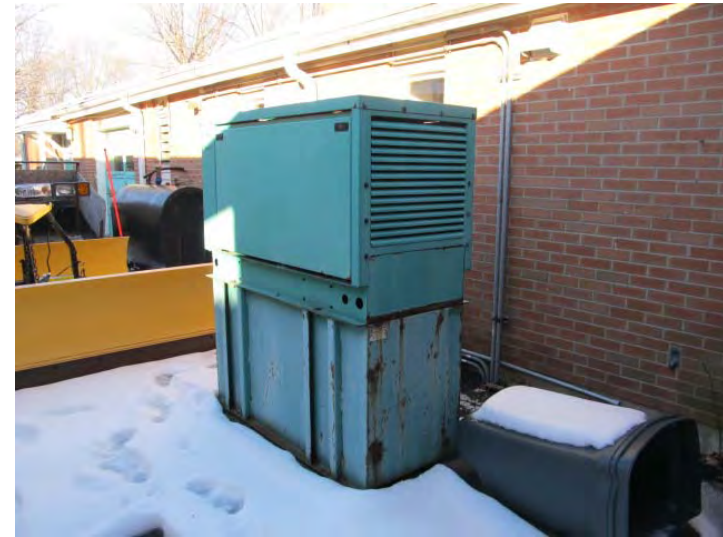
Diesel-fired generator for emergency power at Community Building
