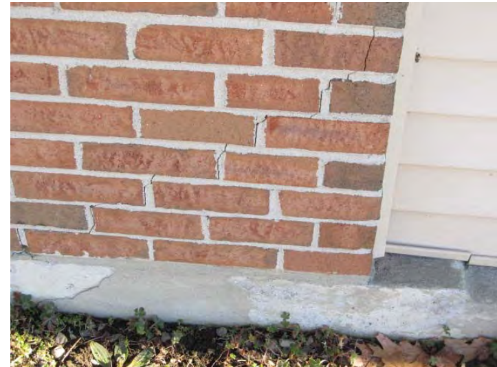
Brick veneer in good overall condition with only isolated minor cracks noted
