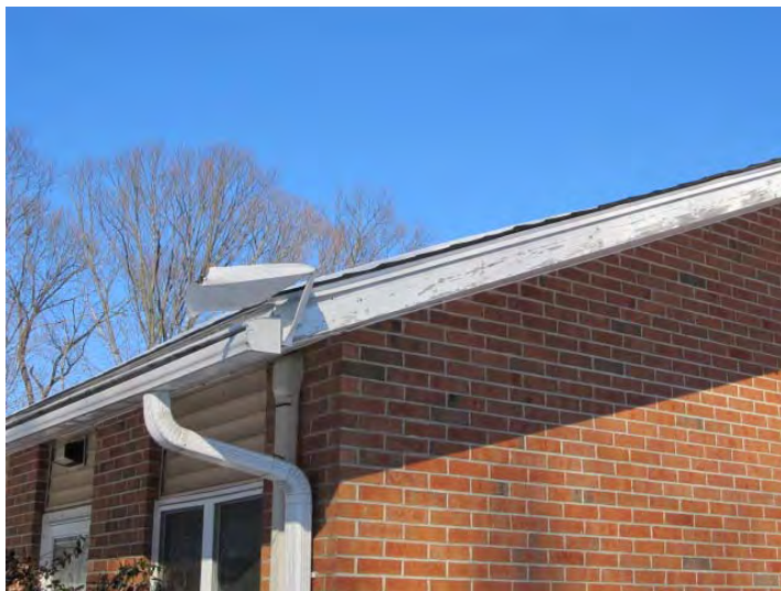
Isolated area of damaged aluminum cladding noted on rake board
