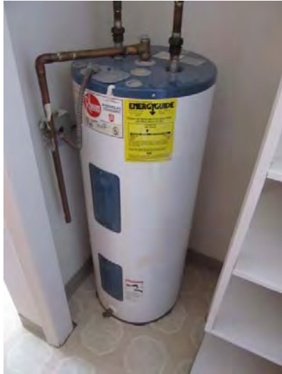
Each unit has its own electric domestic hot water tank – Most tanks currently near or beyond ten years of service
