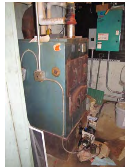
Original oil-fired hydronic boiler for space heating at Community Building
