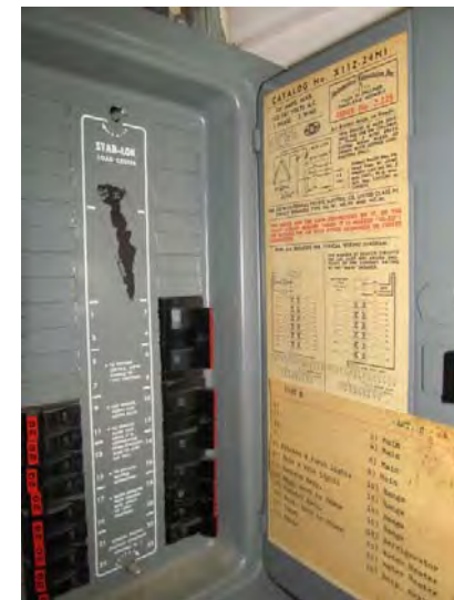
Original 'Stab-Lok' circuit breaker panels by Federal Pacific noted in some units
