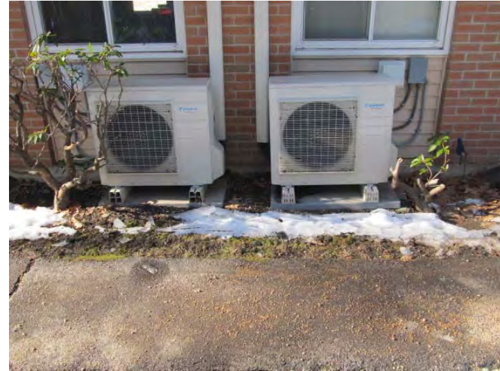
Recently installed exterior condensers for heat pump systems found at all units
