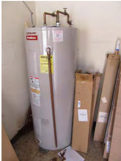
Typical electric domestic hot water tank found at common areas (Community Building and laundry rooms)
