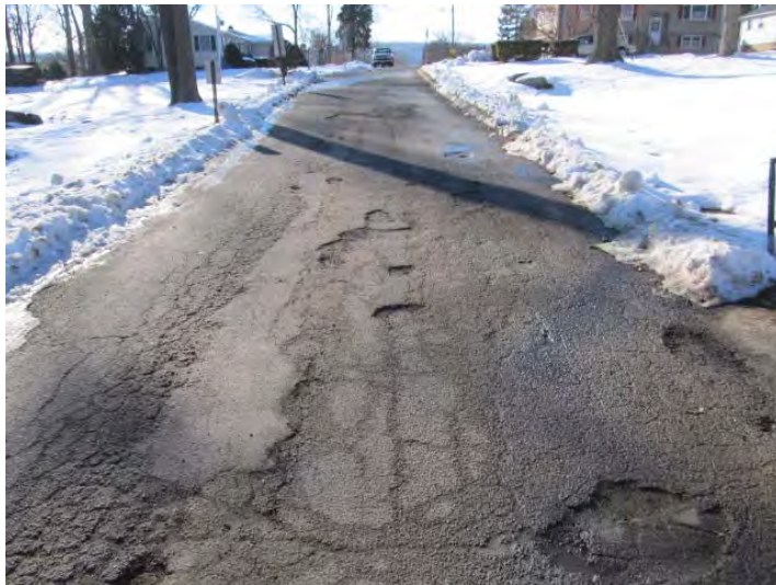
Significant wear/deterioration evident at some asphalt-paved roadway and parking area locations
