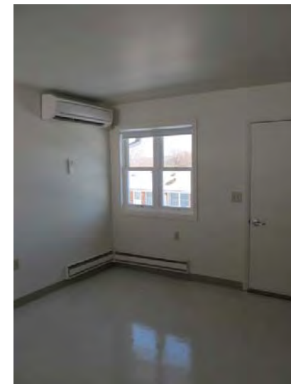
Typical unit interior with vinyl composition tile (VCT) flooring – Note newer wall-mounted component for heat-pump system and original electric resistance baseboard radiation
